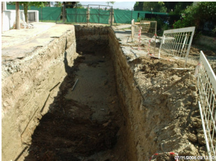
Figure 3. Storm sewer with dead end at boundary between two Municipalities. Photographs taken during storm water sewer construction soon after and few days after rainfall.
