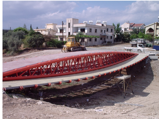
Photograph During Construction
